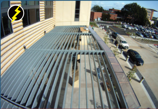
An open steel canopy above an eating area was attracting birds. Constructed from steel beams on their edge the narrow perches were perfect for AVITHOR E-TRACK.
