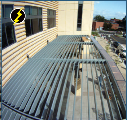
The beams are spaced about 350mm apart. Every top surface was protected
