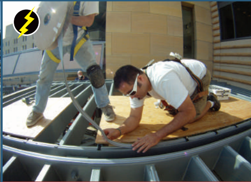
AVITHOR E-TRACK is laid down onto a pre-glued beam. E-Quicks at every intersection facilitated connections to the tracks running down each beam.
