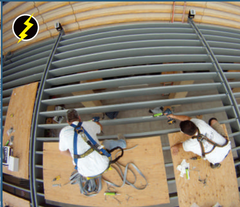
The view from above. Working on thick sheets of plywood, the installers could easily access all the areas to be treated. Notice three of the five chargers mounted on special brackets.
